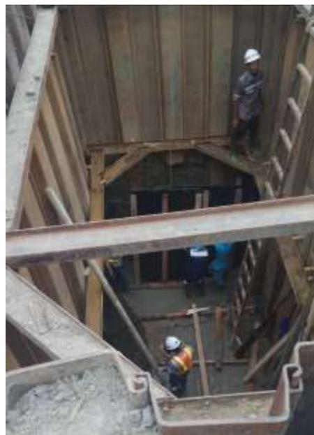
**Figure 7. Starting pit shaft construction on Jl. Sidorukun.**
