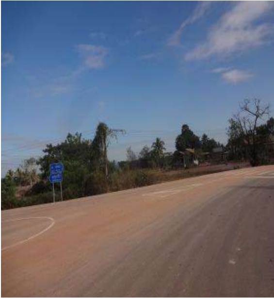
Plate 1: Completed asphalt paved new access road along the flood embankment subproject
