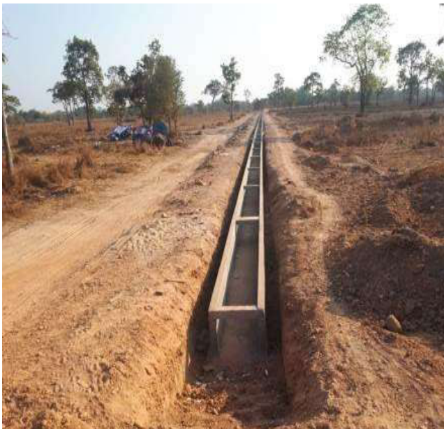
Plate 7: A lot of ground restoration and clearing operation that needs to be done yet along the canals in the irrigation subproject
