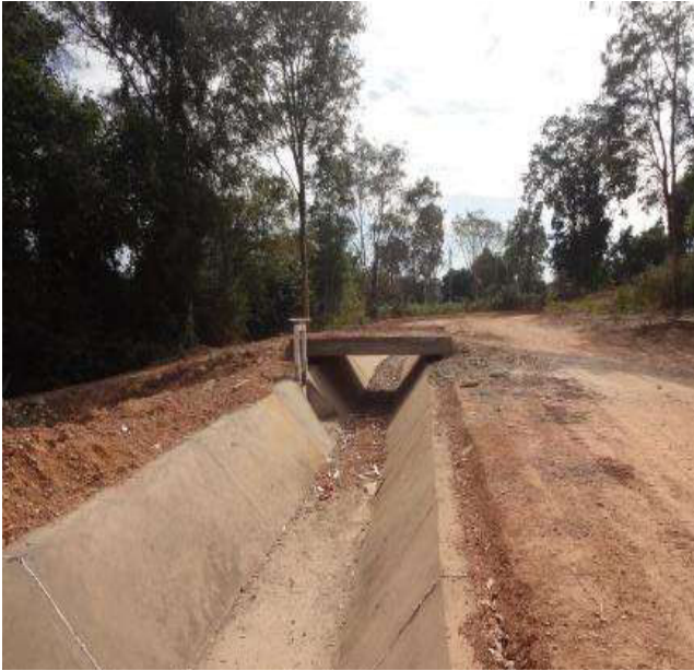
Plate 5: Almost completed primary irrigation canal at Donkhuay Irrigation Scheme
