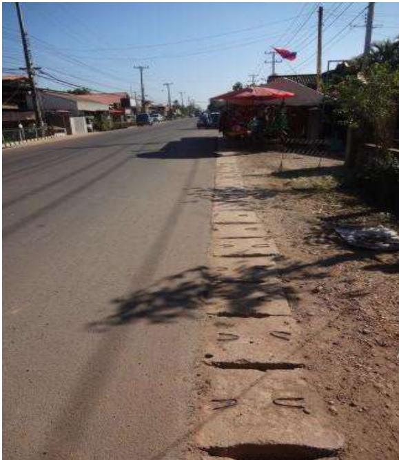
Plate 3: Completed concrete drainage along the road-dike
