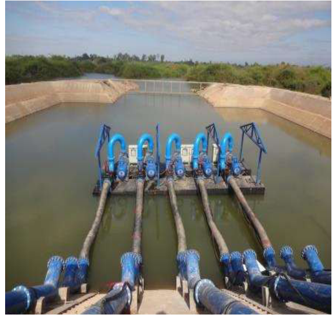
Plate 6: Newly installed water pump at Mak Hiao River
