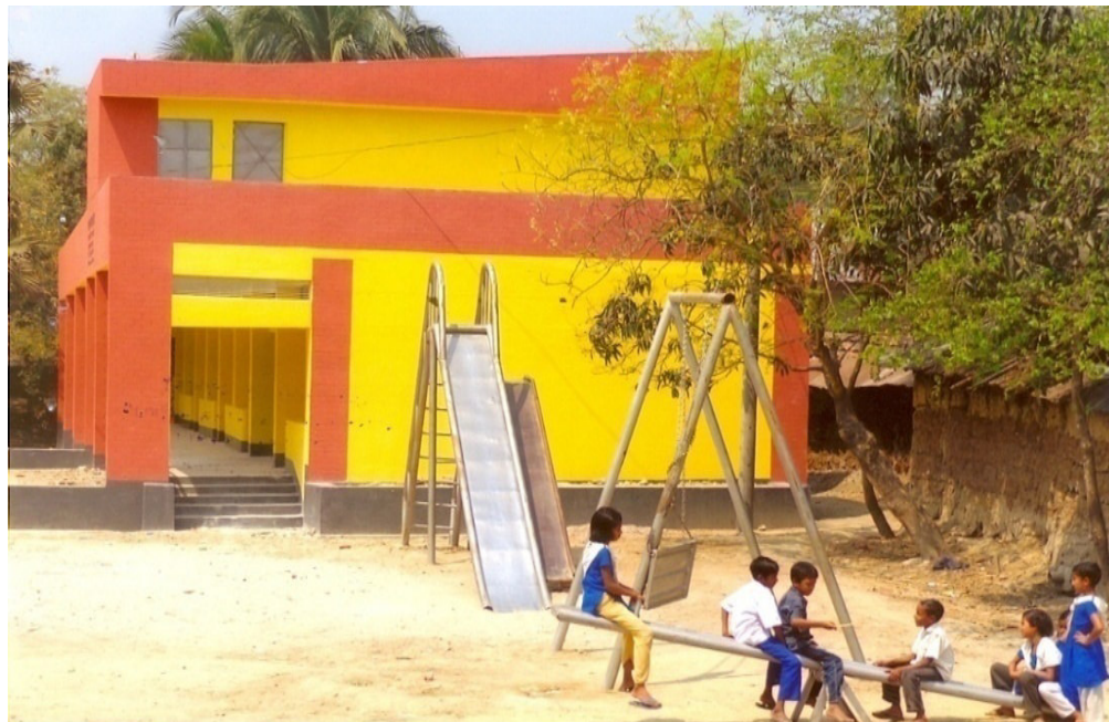
Fig 2 Children Park adjacent to school building
