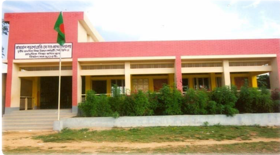
Fig 1 Plantation in PEDP 3 school building
