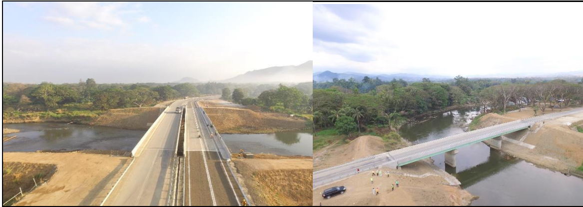
Photo 2 Laloki Bridge Site preparation for planting grasses & trees
