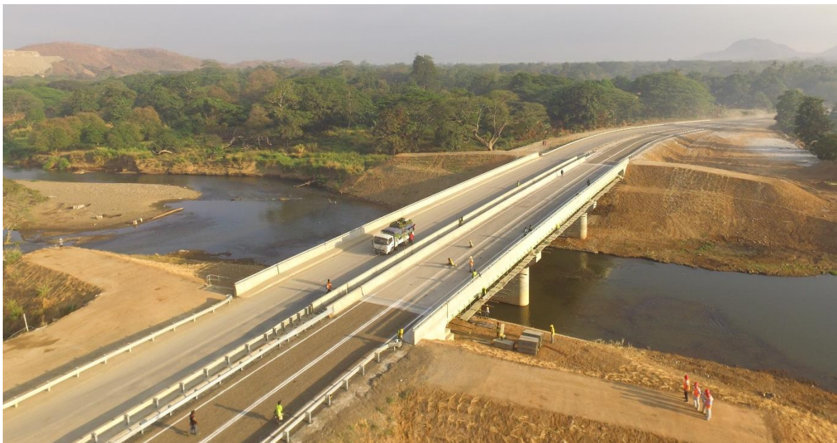
Photo 4: See Natural water quality at Laloki immediately after construction.
