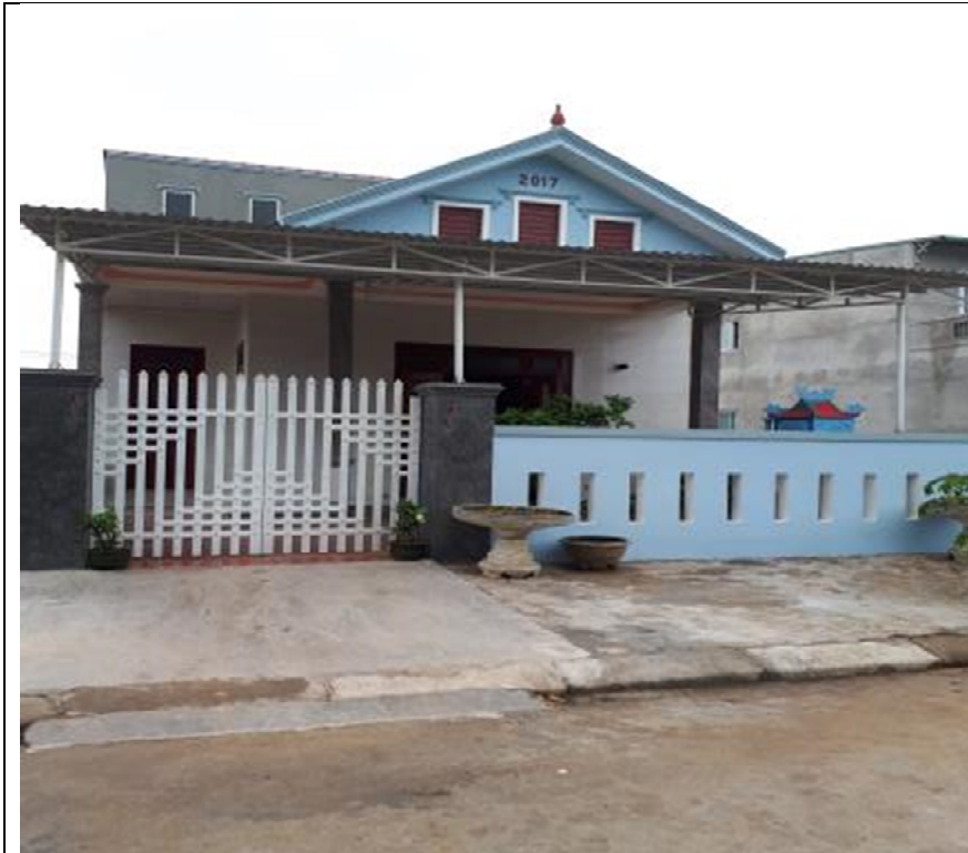
An AH moved and built new house onto Group 6, Dong Le Ward Residential Site
