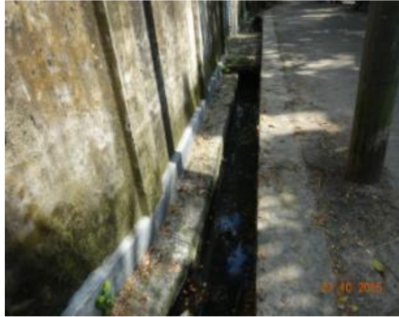
Existing condition of SD-13
