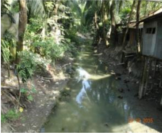
Existing condition of SD-12
