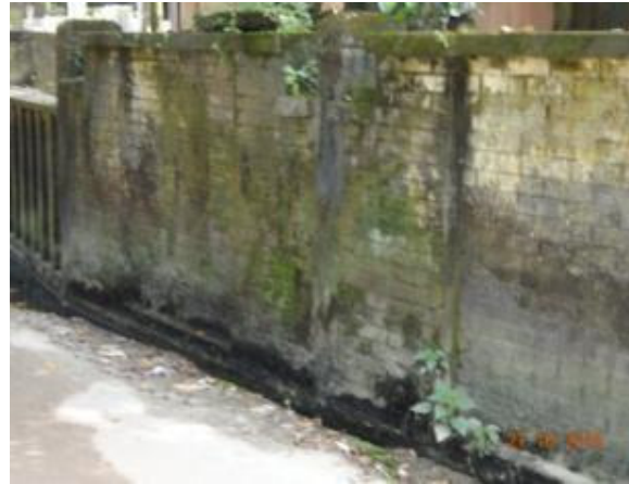
Existing condition of SD-07
