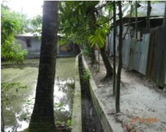
Existing condition of SD-06
