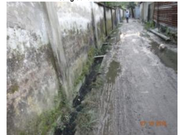
Existing condition of SD-11
