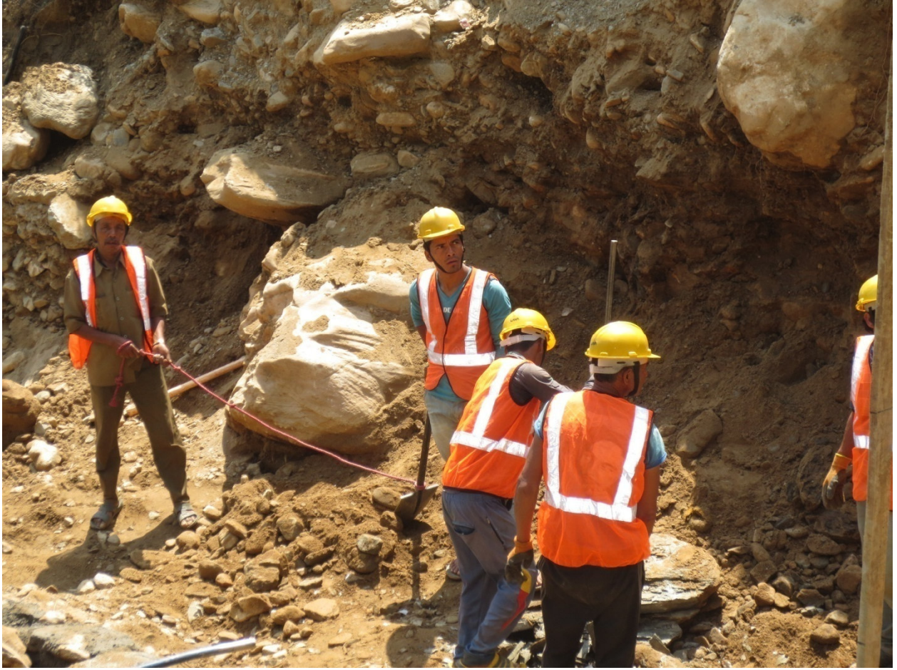
Construction at Simrutu khola mini hydro sub project
