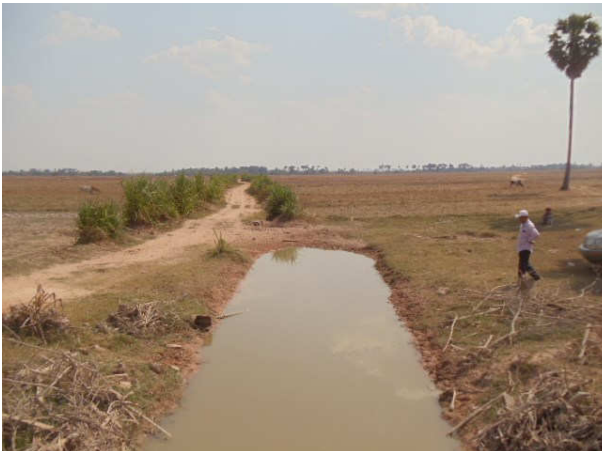
Photo 1 Proposed Canal Looking Upstream Location Condition
