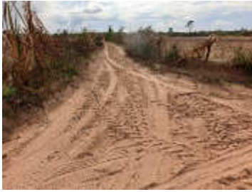
Existing condition of 8 meters of oxcart road
