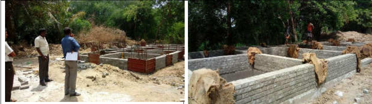
Kankodutha Vanigam (Resettlement site) site inspection by the PMU
