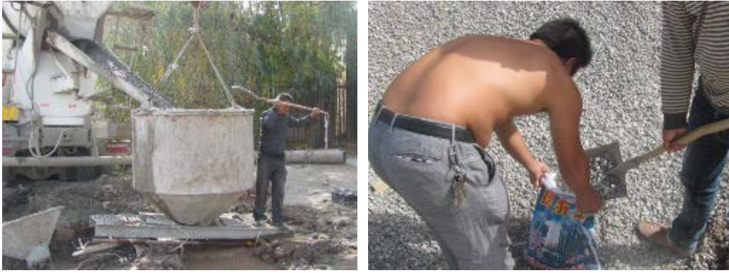
Figure 4-1 Participate in the project construction villagers
