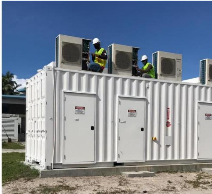
**Figure 4. a/c installation in Addu BESS**
