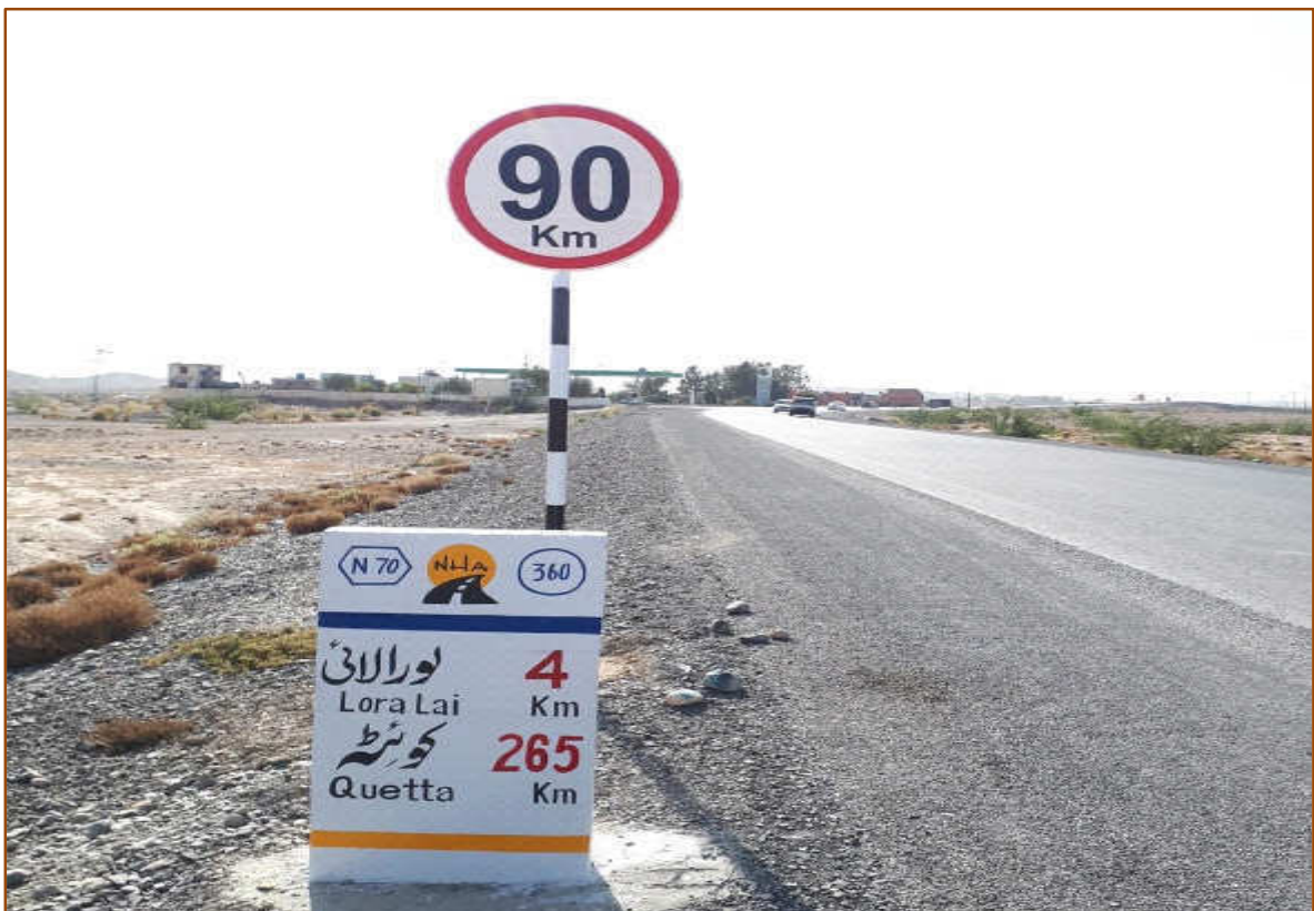
Picture 4: Completed Road Section Lot-2
