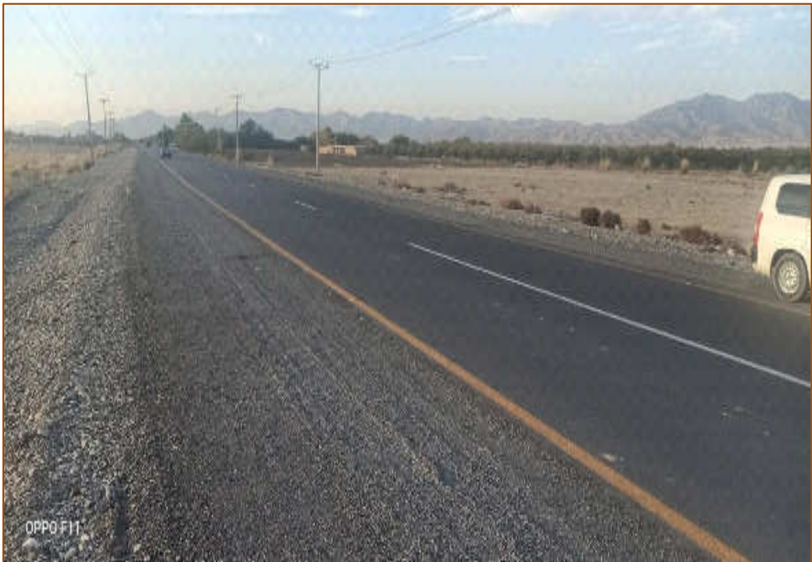
Picture 3: Completed Road Section Lot-1
