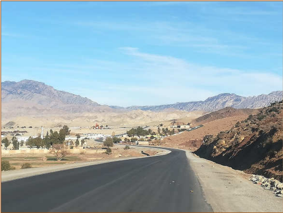
THE COMPLETED SECTION OF ROAD AT LOT-1
