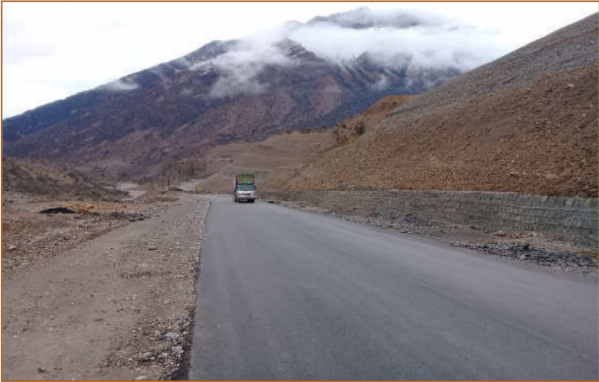
THE COMPLETED SECTION OF ROAD AT LOT-2
