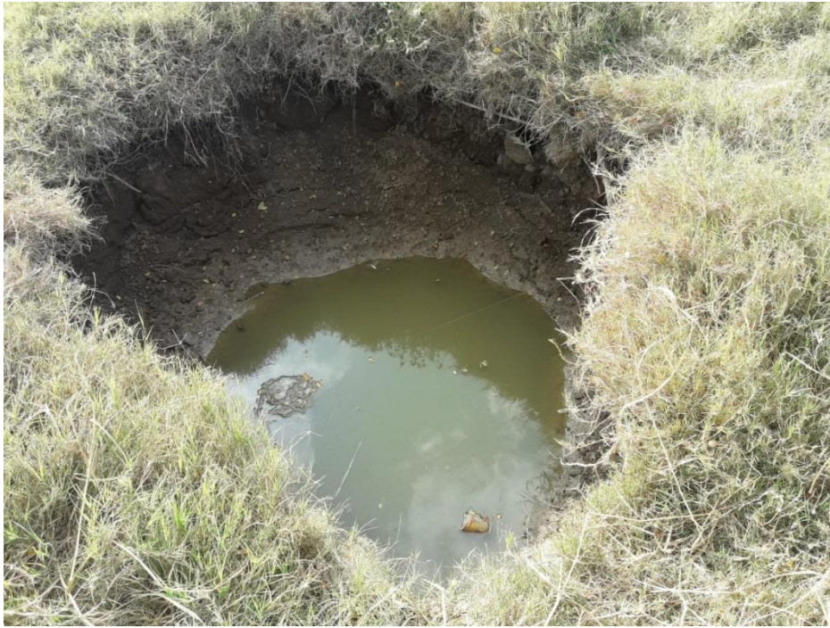
Figure 1: Existing surface well used for pumping water
