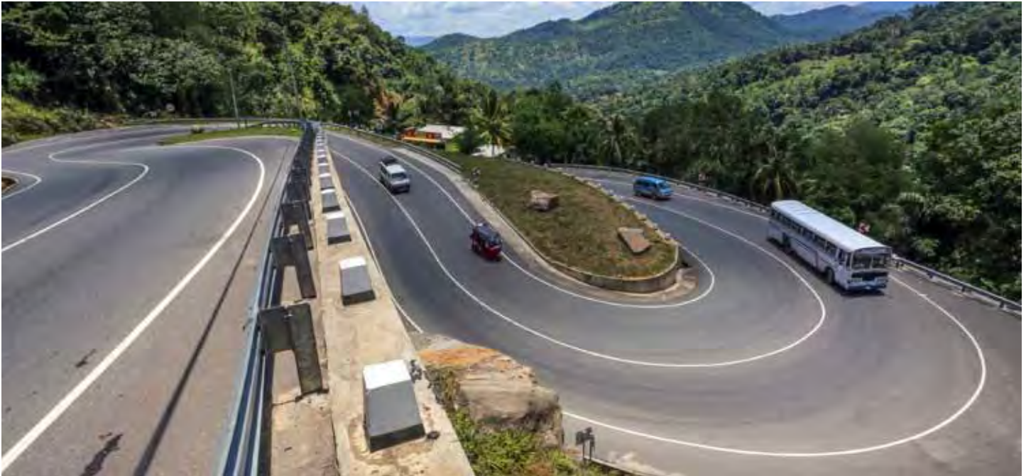
The Kandy-Mahiyangana national highway in central Sri Lanka was upgraded under the ADB-supported National Highways Sector Project.
