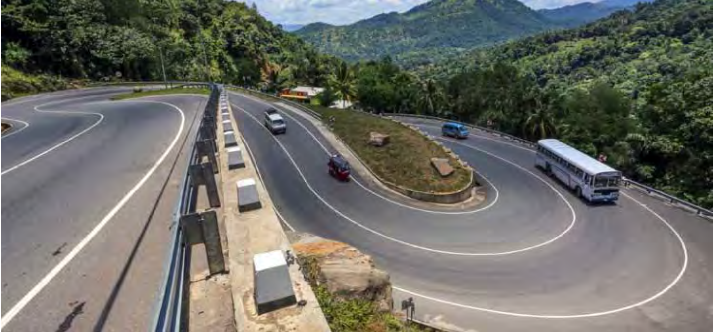
The Kandy-Mahiyangana national highway in central Sri Lanka was upgraded under the ADB-supported National Highways Sector Project.
