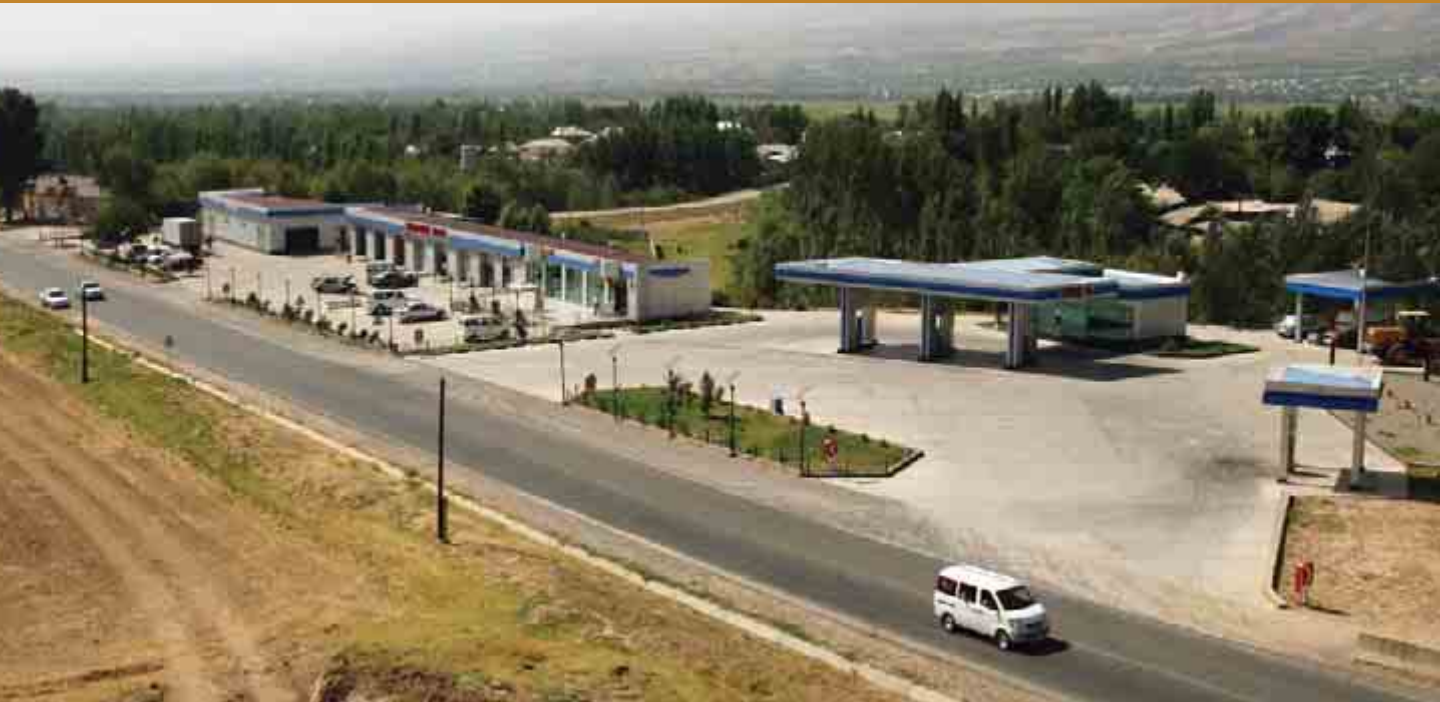
Roadside facility, Dushanbe–Kyrgyz Border Road Rehabilitation Project (Phase III)
