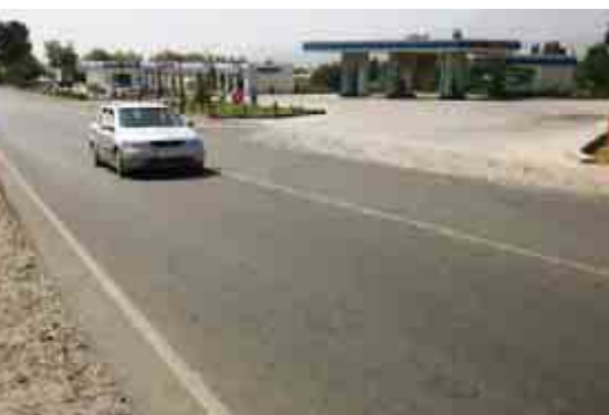
Vahdat district, Dushanbe–Kyrgyz Border Road Rehabilitation Project (Phase I)
