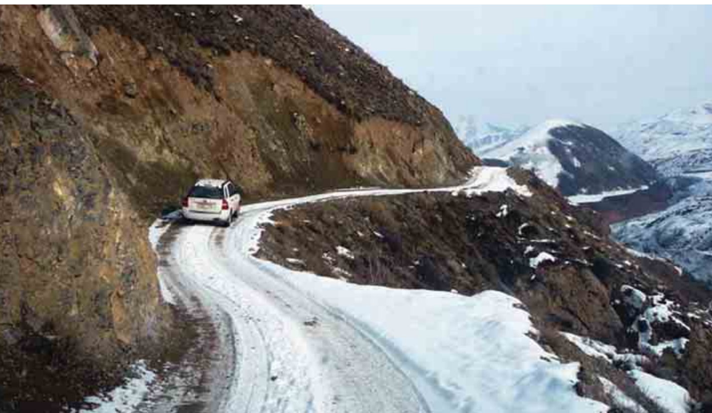
Karamyk section before improvement, Dushanbe–Kyrgyz Border Road Rehabilitation Project (Phase III)
