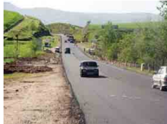
Km 33+500, Dushanbe–Kyrgyz Border Road Rehabilitation Project (Phase II)
