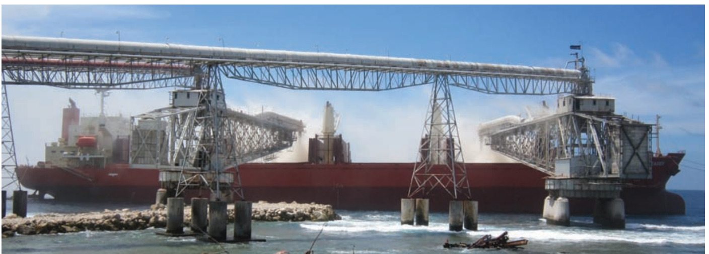
Cantilever loading phosphate onto a ship for export at RONPHOS headquarters
