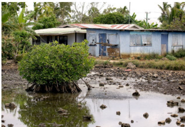
Houses built in a flood prone area, Popua village, Nuku'alofa, Tonga
