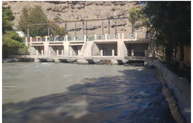
Chubek Canal main gates. The gate controls inflow from Pyanj River to Chubek Irrigation System (photo by Project Implementation Group, Agency for Land Reclamation and Irrigation).
