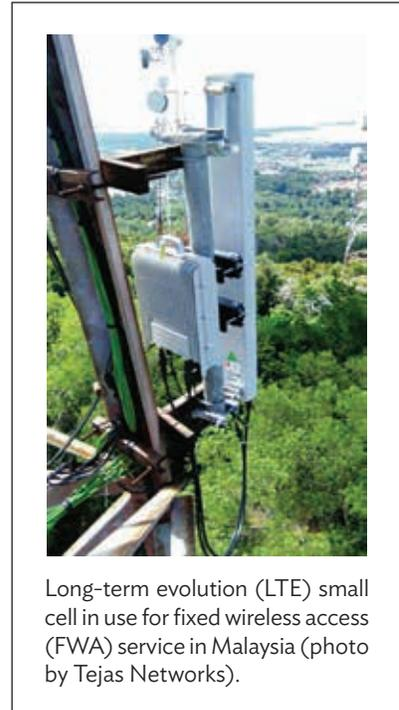
Long-term evolution (LTE) small cell in use for fixed wireless access (FWA) service in Malaysia (photo by Tejas Networks).
