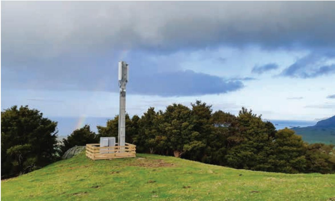
This small multi-operator core network (MOCN) tower, located at the Whangarei Heads in New Zealand, allows three carriers to share equipment and radio spectrum to provide long-term evolution (LTE) in the 700 MHz band to a remote location (photo by Rural Connectivity Group).
