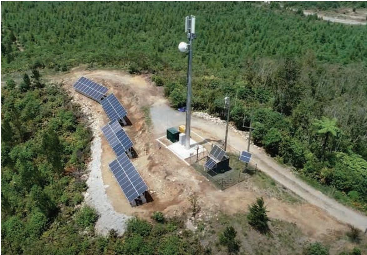
This shared rural LTE tower has three sectors and one microwave backhaul link. Supporting it requires a large solar array plus a diesel generator. Energy requirements take up more than 100 square meters of land (photo by Chris Parker. RCG at TECT Park Cell Tower, 2021. [https://www.youtube.com/watch?v=9LlgH\\_mp2d4](https://www.youtube.com/watch?v=9LlgH_mp2d4)).
