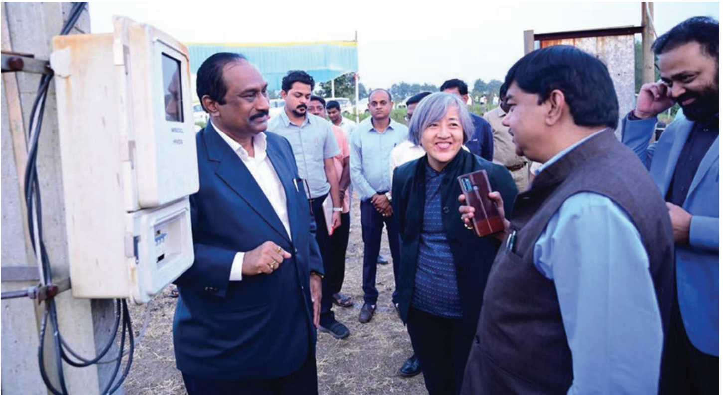
Site visit. The project team, with ADB Executive Directors Chantale Wong and Sameer Kumar Khare, inspect one of the low-capacity distribution transformers installed by the project in Maharashtra.
