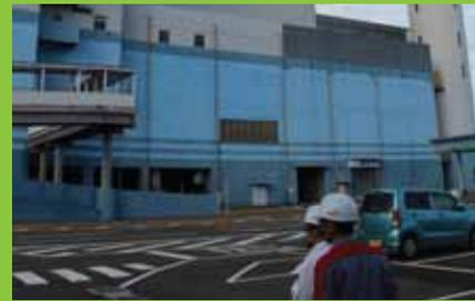
Incinerator Facility is focused on recycling waste by combusting refuse at high temperatures. Thermal energy generated during refuse treatment is utilized for electric power generation that is reused in the facility, as well as sold to the local private utility company.
