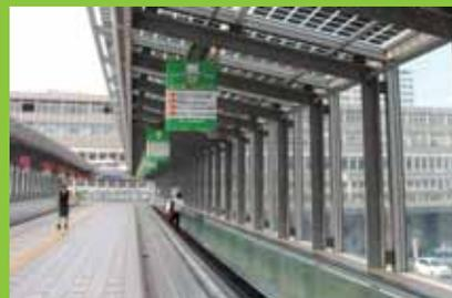
Solar panels are integrated in walkways to increase the production of electricity from renewable sources.
